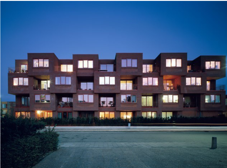
Image 8.7: Nighttime view of the northern facade. There is a large open field on this side of the building.
