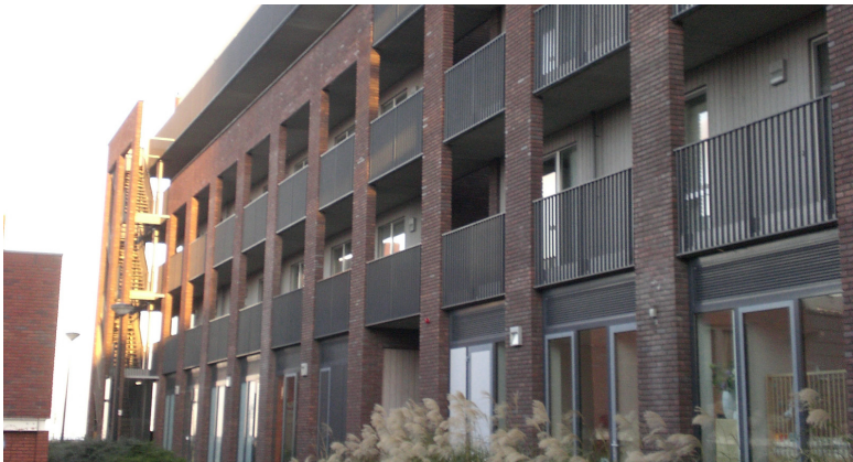
Image 2.5 : Block 25 C back facade source: website of Faro Architecten
