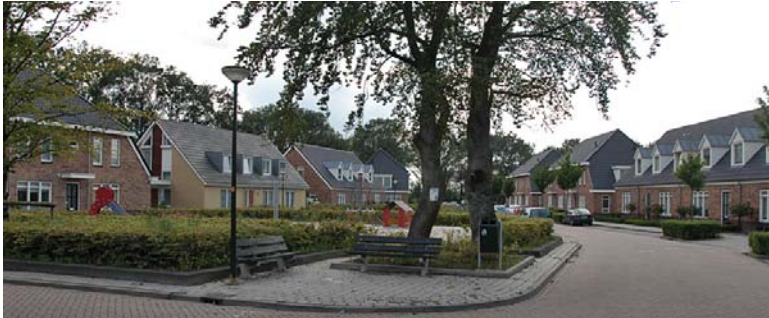
Image 12.1: General View to the Site Source (of all the images): Official Website of "Van Den Pauwert Architecten"
