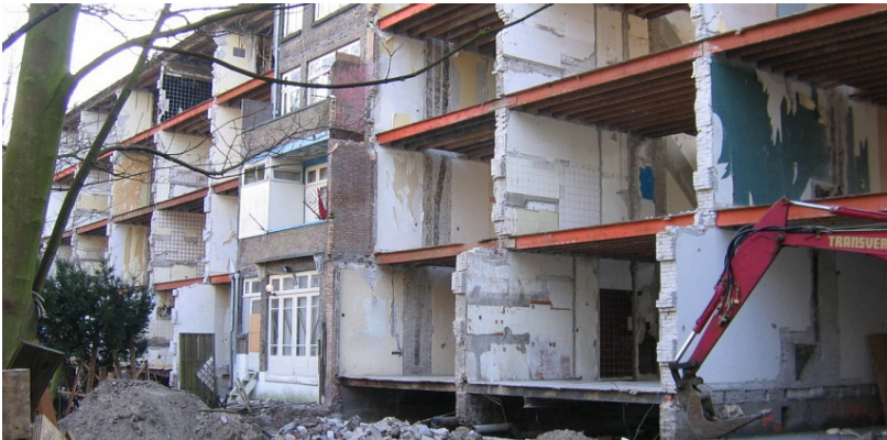
Image 15.2: Facades after being demolished for renovation
