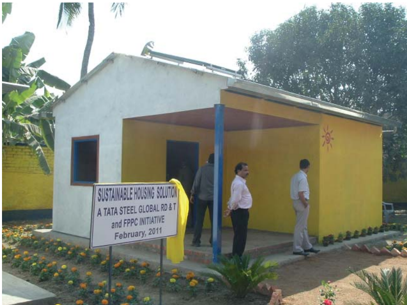
Image 18.1: Tata Nano House in testphase (Frontside) source image : Tata Steel
