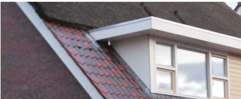
Image 11.3: Detailview thatch roof with roof tiles
