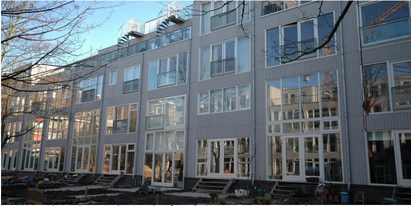
Image 15.1: General view to the site taken from the inner common courtyard Source (of all the images): website of Hulshof Architects
